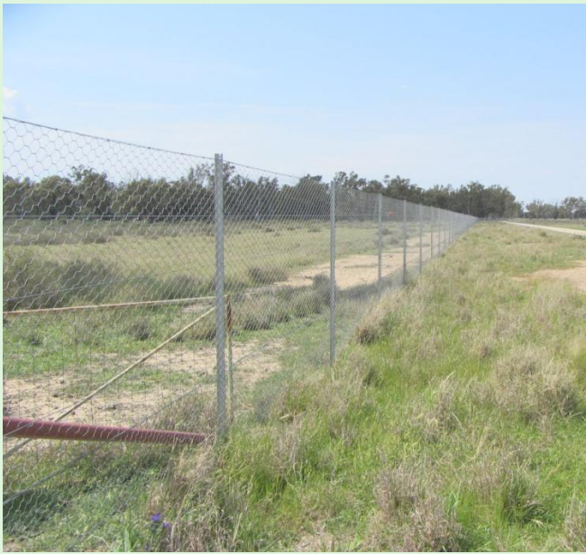
Figure 7: 2m high fence around 20ha soft release enclosure at Moulamein in the Riverina.
